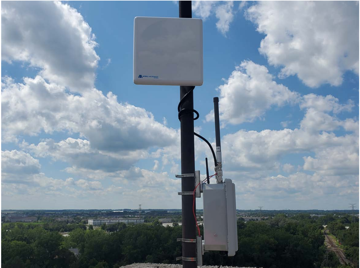
FOAM radio "build-it-yourself" version, installed on a mast above a building in Illinois.
